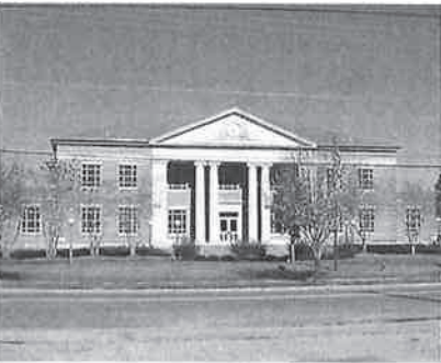
Baker County Courthouse Restoration
