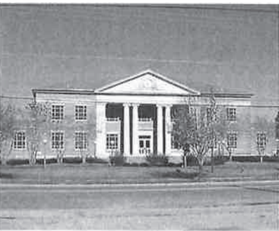
Baker County Courthouse Restoration
